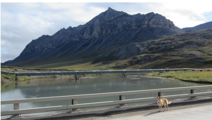
Crossing the Atigun River. Photo looks east.
